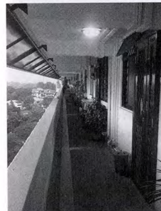
HOUSING AND DEVELOPMENT BOARD ESTATE GHIM MOH, CONSTRUCTED IN THE EARLY 1970S AND RETROFITTED IN THE 1990S, SINGAPORE, 2011. TOP: HOUSING AND DEVELOPMENT BOARD ESTATE GHIM MOH, SINGAPORE, 2011. PHOTOS: CARY SIRESS.
