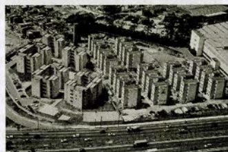
AERIAL VIEWS OF CINGAPURA HOUSING PROJECTS, SÃO PAULO, 2012. PHOTOS: FERNANDO STANKUNS & FABIO KNOLL.
