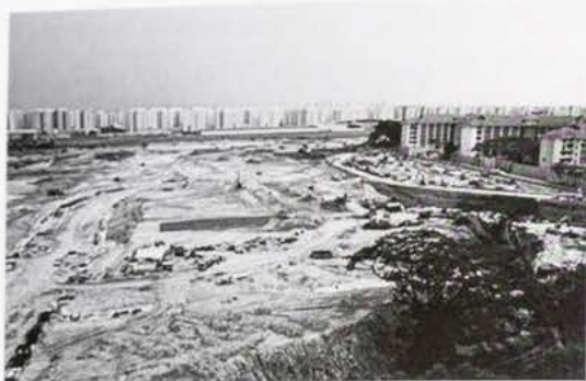
CLEARED SITE AT BUANGKOK (SOURCE: SINGAPORE HARDWARE ZONE FORUM, 2016)
