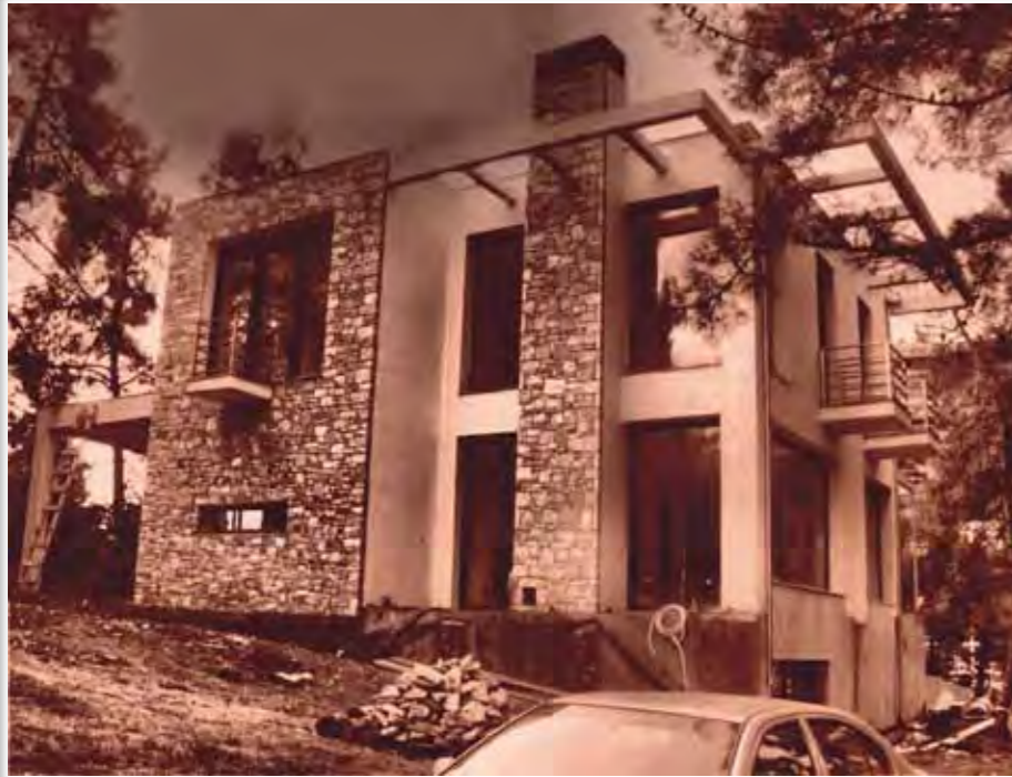
Building under construction
