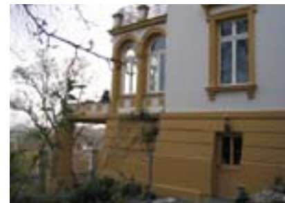
Sockel Sockel in Hanglage
