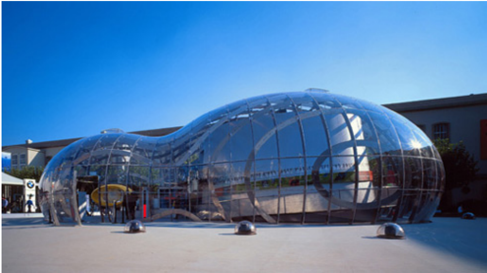
Bernhard Franken: Bubble, Frankfurt, Germany, 1999 form as metaball simulation of water drops
