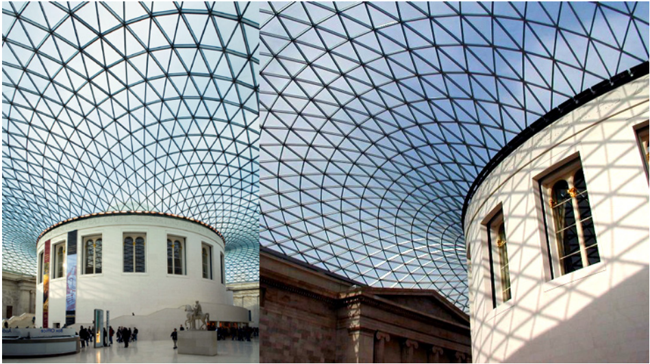
Norman Foster and Partners: Great Court Roof, British Museum, London, UK, 1999-2000 geometrically defined parametric model based on algebraic overlay of three surfaces; shape optimisation by method of relaxation
