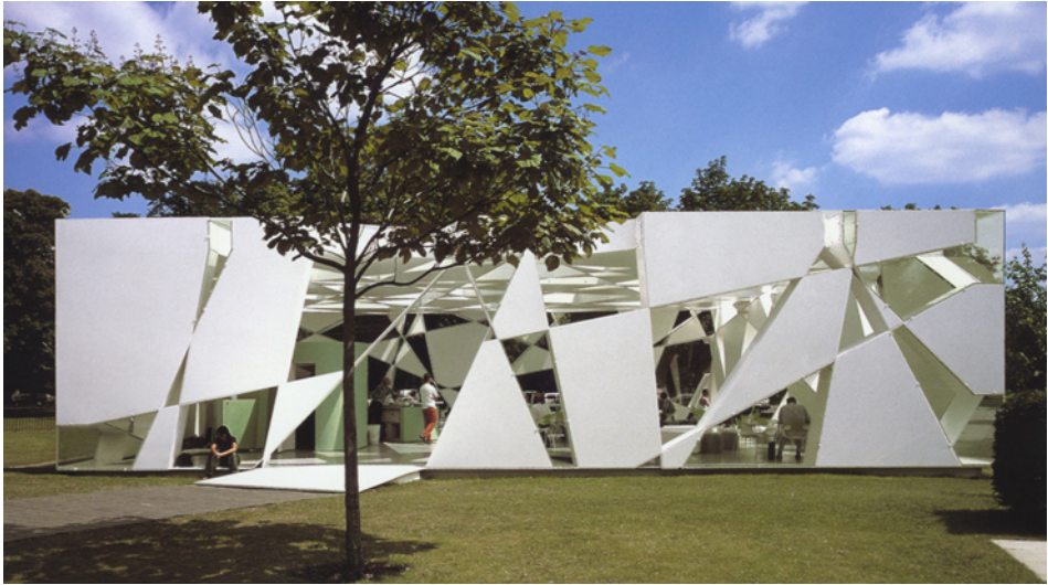
Toyo Ito: Serpentine Gallery Pavilion, London, UK, 2002 complex weave out of repeated nesting of rotated squares and extension into field of intersecting lines
