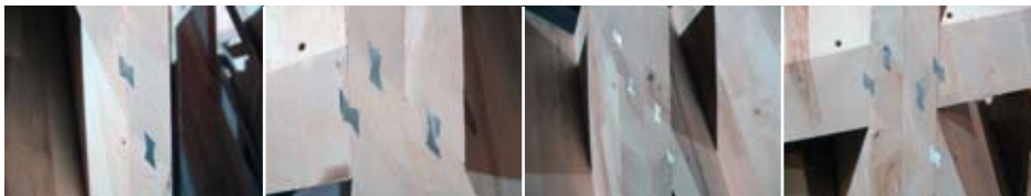
The parts of the sculpture are connected with aluminum dovetails. Sloped cuts through the dovetails result in interesting geometries.
