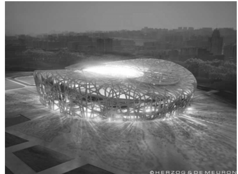
national stadium beijing
