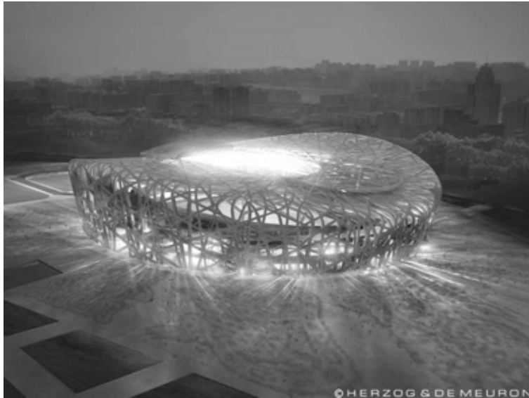
national stadium beijing
