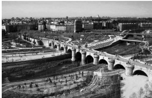
Fig. 17 Connections: the new Madrid Rio park brings previously divided neighborhoods together and facilitates multiple episodes.
