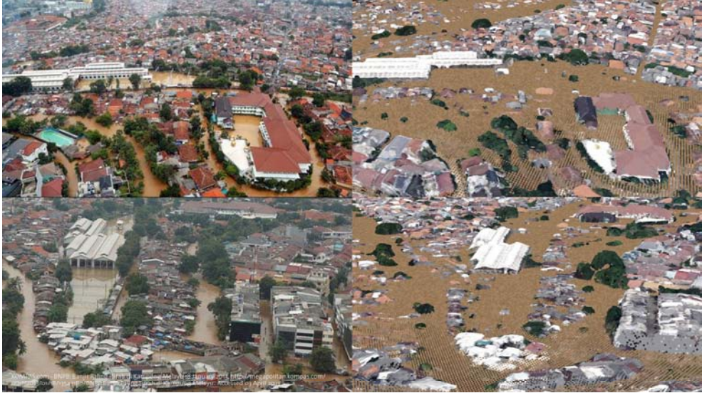
Fig. 5: Left: Photographs of flooding in 2013. Right: Visualization of a flood simulation run through the same sites within the point cloud models. Landscape modifications can be embedded in the point cloud model and then events simulated to compare against this base case.
