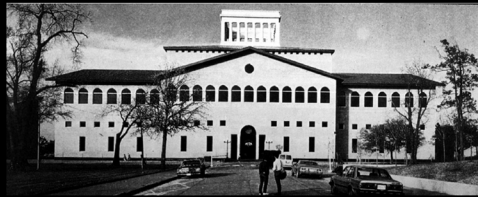
Claude-Nicolas Ledoux, Perspektive Haus / J. Burgee u. P. Johnson, School of Architecture, Houston Texas, 1982-85
