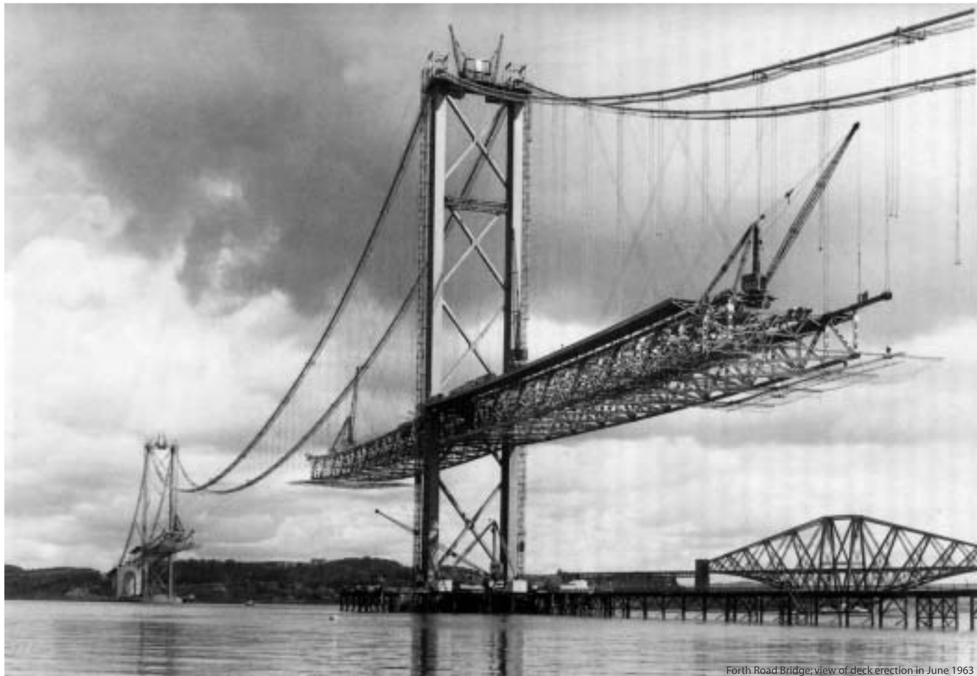
Forth Road Bridge; view of deck erection in June 1963
