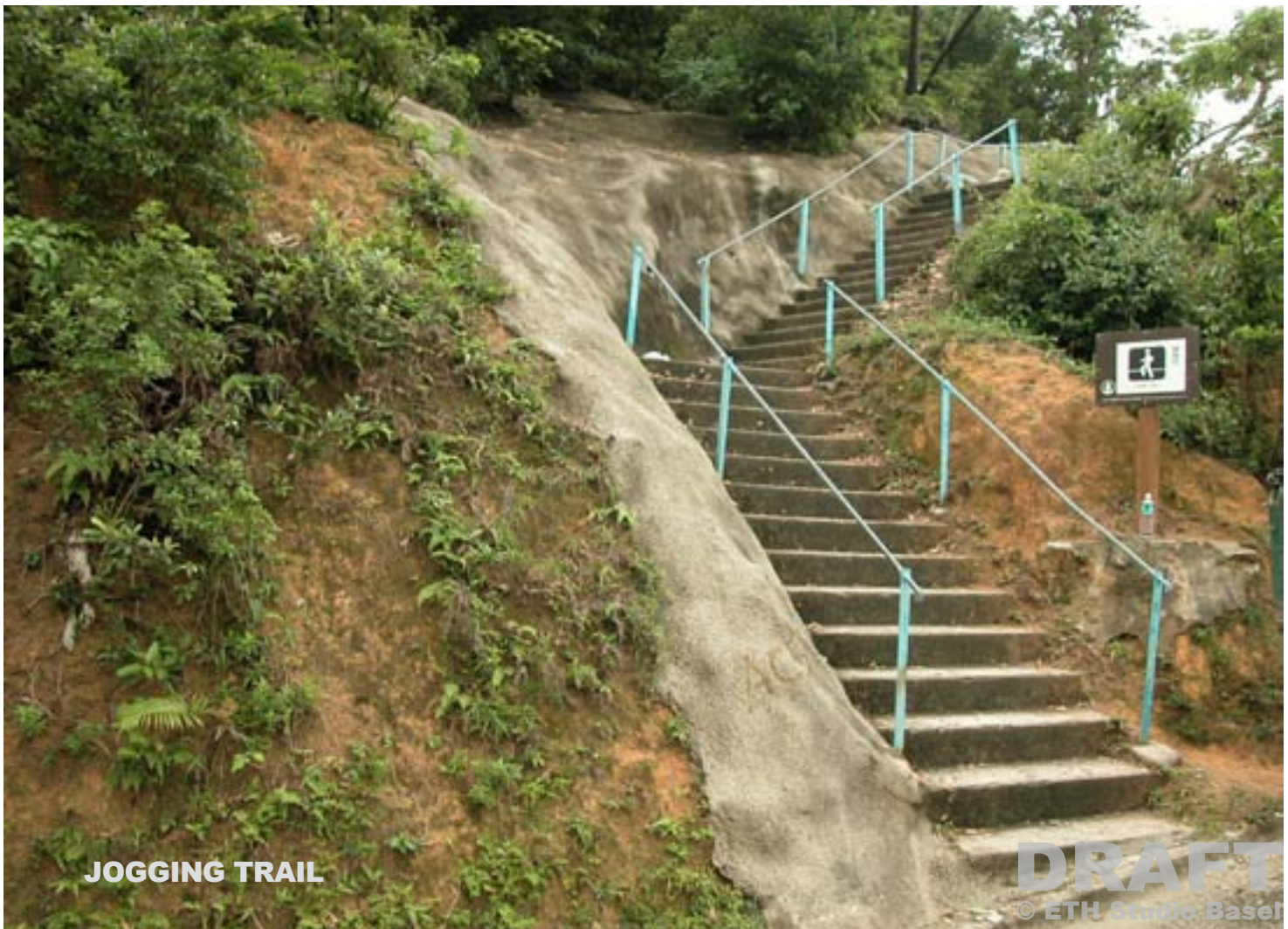
JOGGING TRAIL USED FOR CATCHWATER MAINTENANCE
