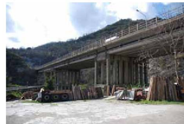
Bridge in Acquasanta Terme
