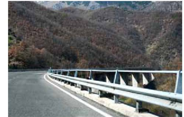
Bridge after exit for Micigliano
