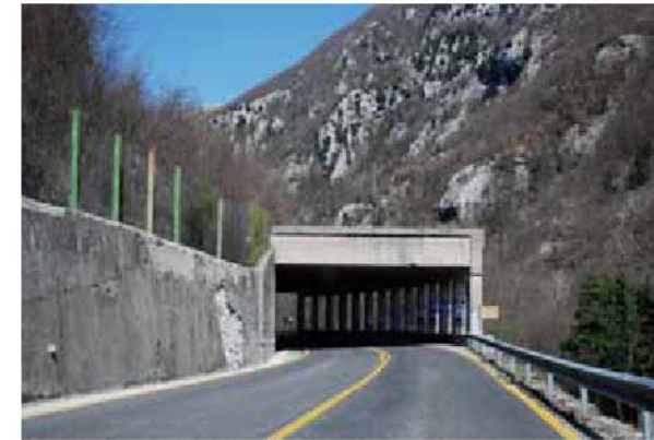
Tunnel after exit for Micigliano
