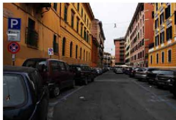
High and dense buildings along via Salaria, creating a "barrier" on the sides
