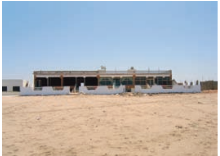
New house under construction
