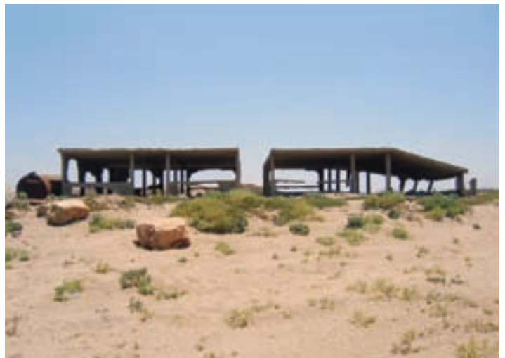
Neighboring house ruined for illegal construction
