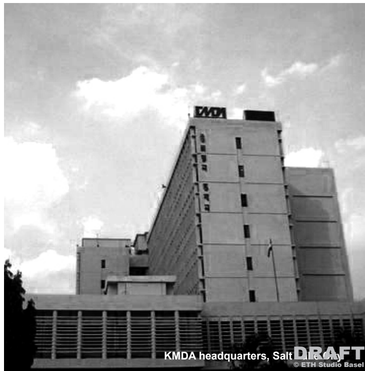
KMDA office building, Salt Lake City
