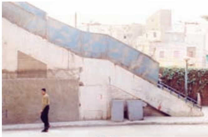
POLICE STATION_BEFORE UPGRADING
