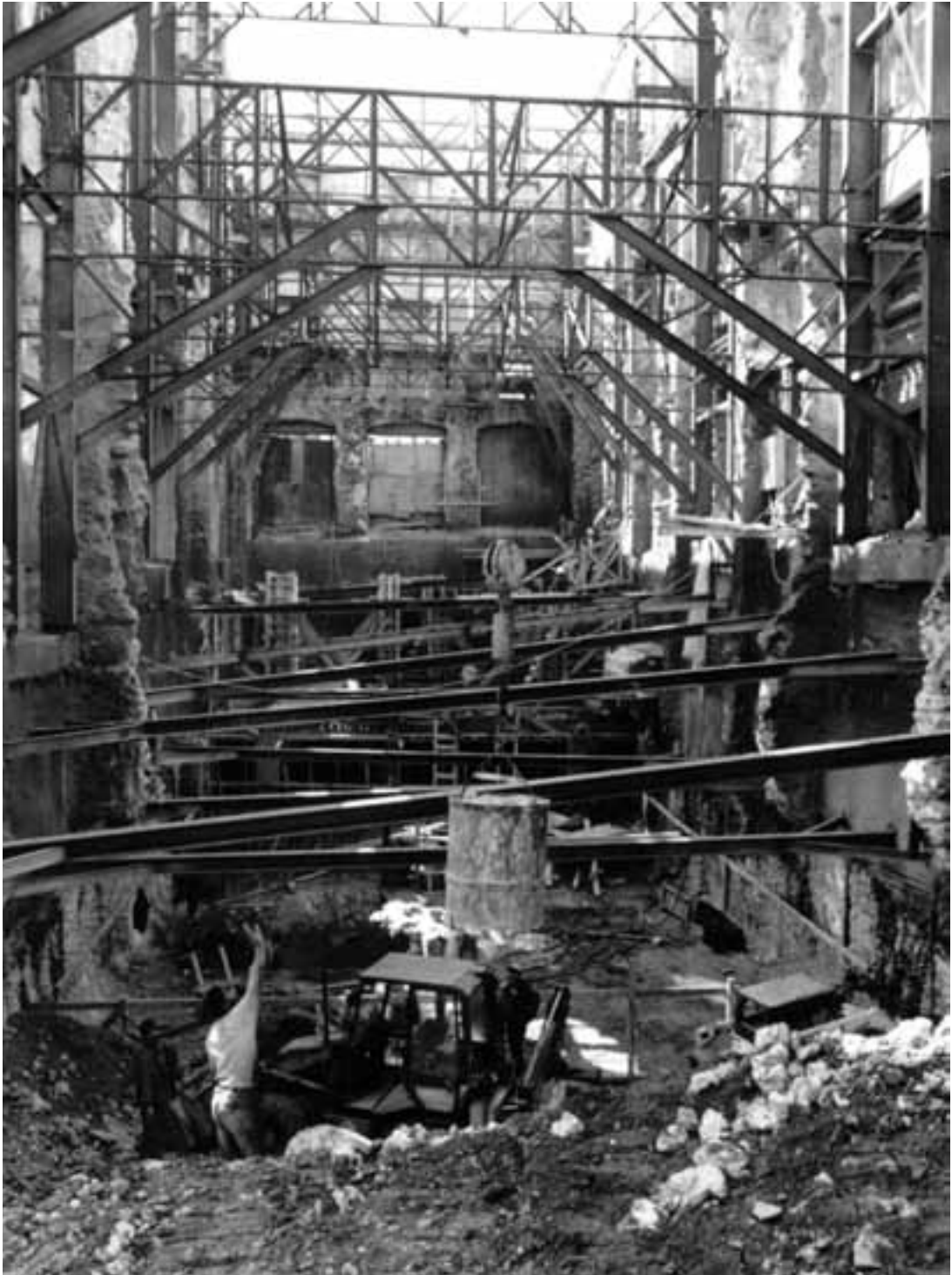
Reconstruction of the Sabbaq building. 1997
