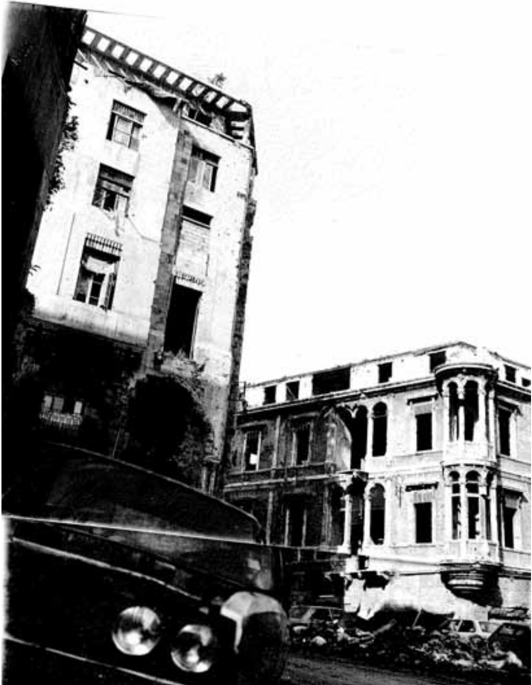
The Audi Bank in its original position. 1991
