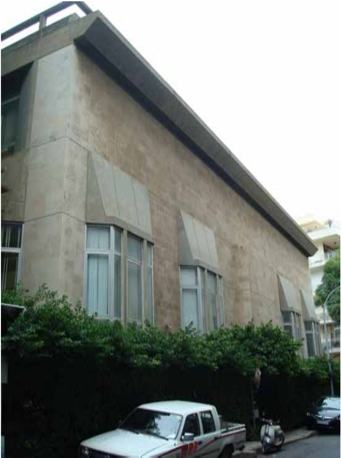
The extension to the back of the Sursock Museum, done in the 1960s. 2009
