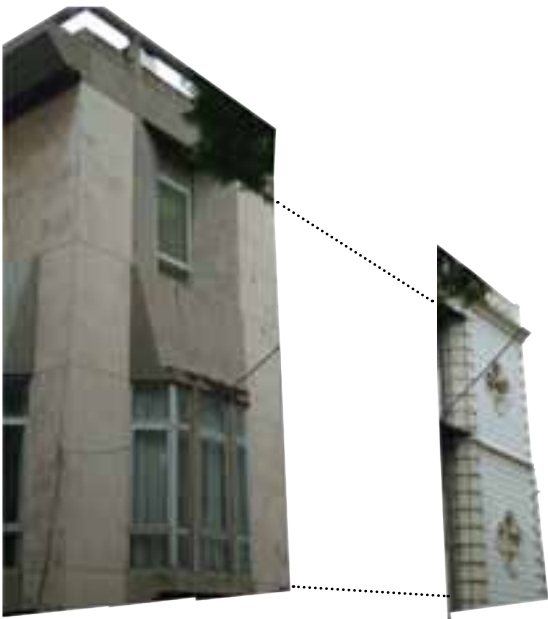
The building appears as schizophrenic with two distinctly different facades
