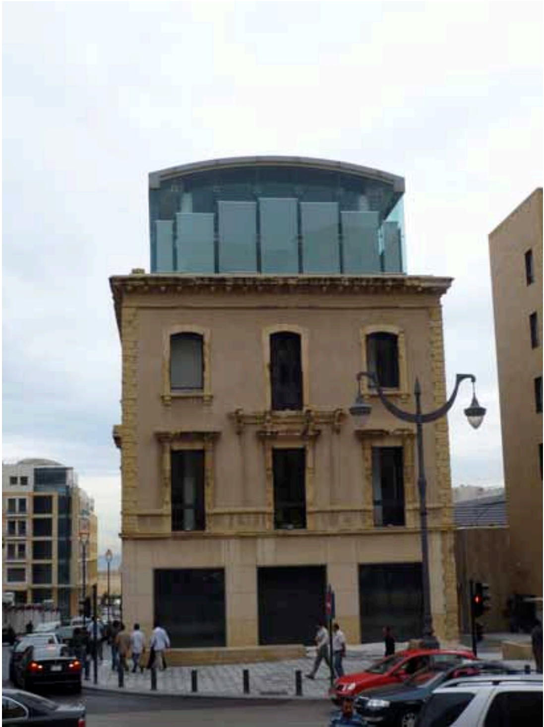
The Sabbaq building. 2009
