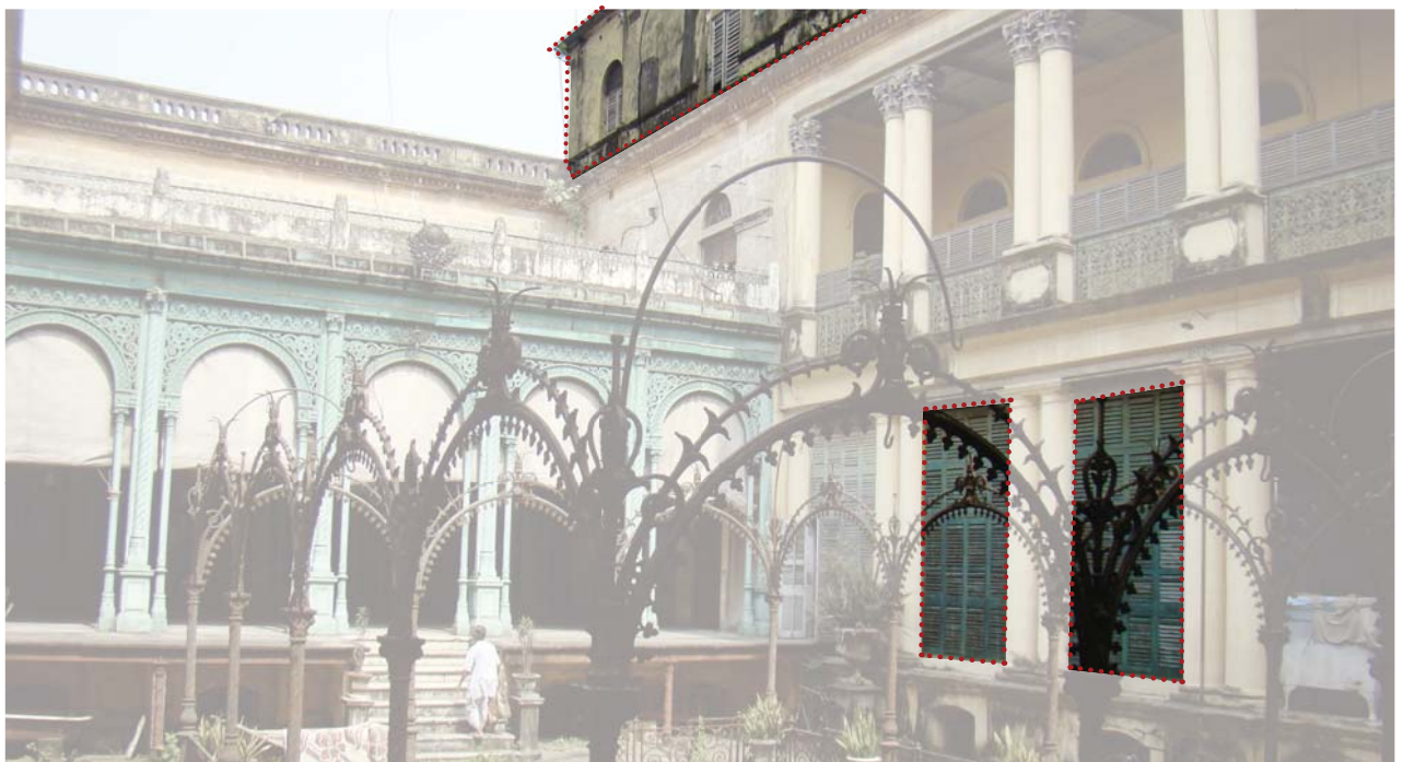
New Addition on Rooftop and New Arcade Partitions
