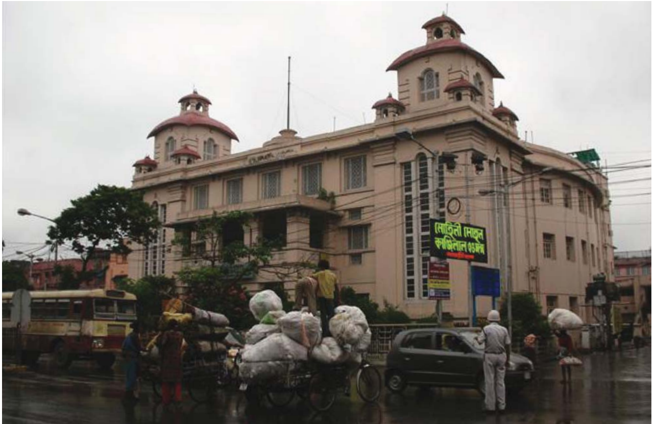
National Radio Hall, Maidan Built: 1960's
