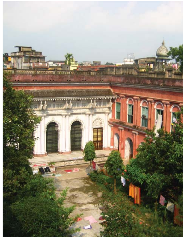
House Exterior and Surrounding Buildings
