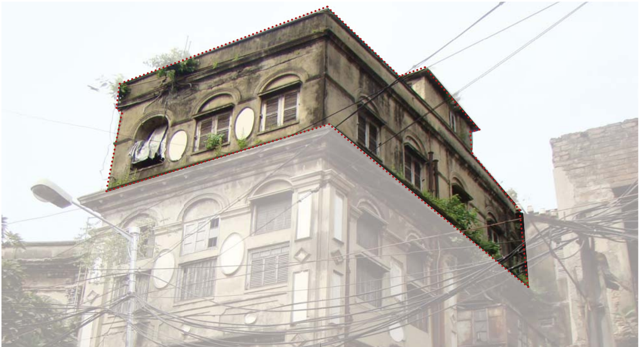
New Rooftop Addition
