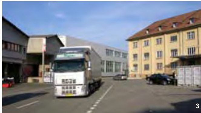
A new university campus for the faculty of art and design of the FHNW will be realised in the Dreispitz-Areal.
