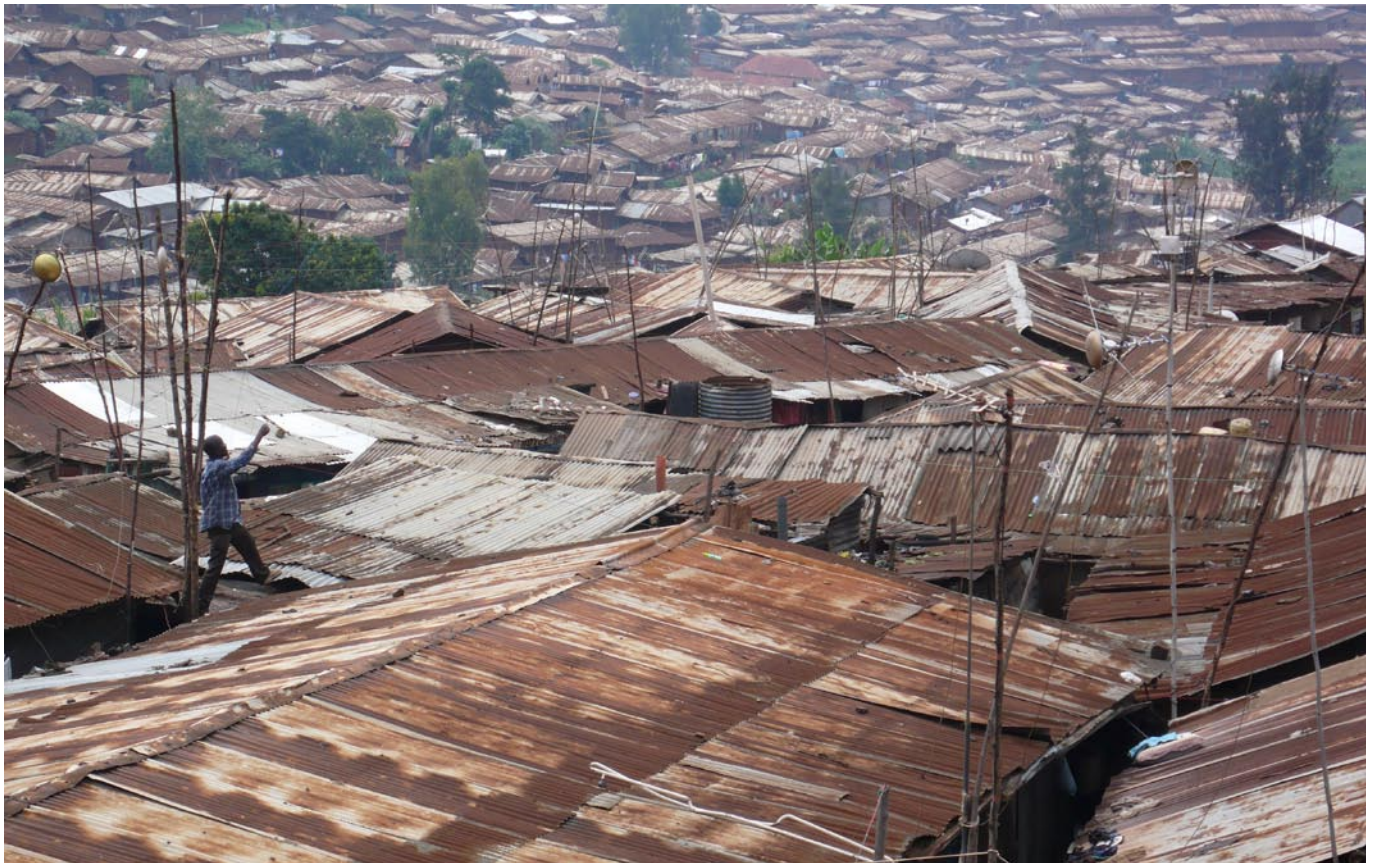
View over the roofs of Kibera
