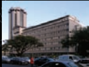
4 Shell and BP House
