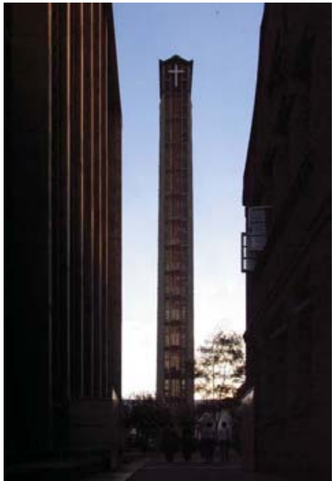
Left Bottom: Interior of the bell tower Right: East Elevation of the bell tower
