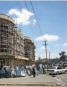
construction of new buildings
