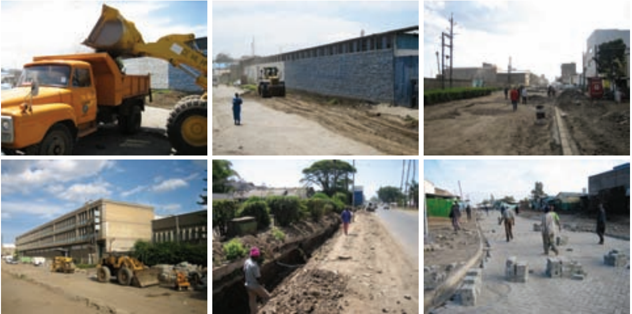
current roadworks of the Nairobi City Council on different streets
