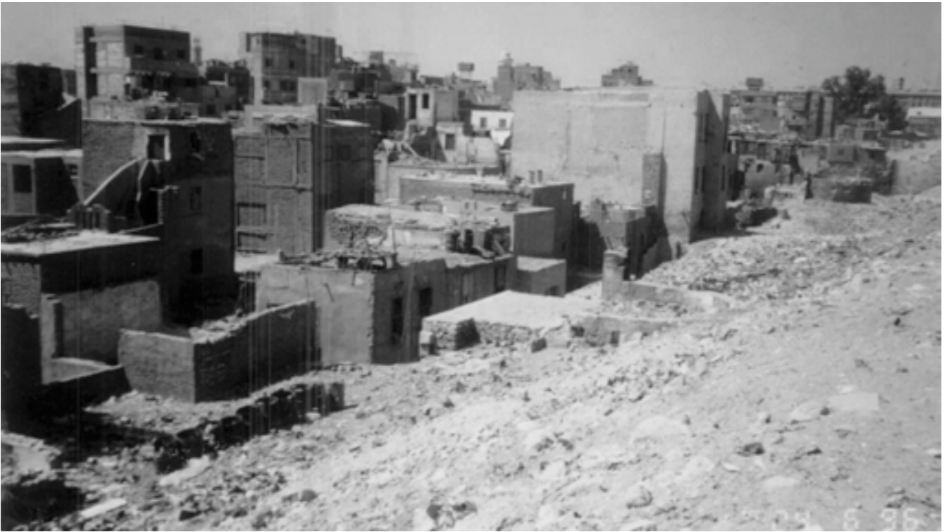
1 The historic Ayyubid wall covered with garbage. Photo: 1996
