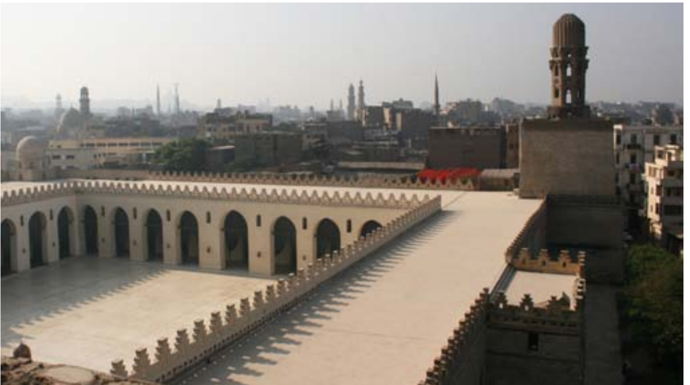
2 Al-Hakim Mosque, destruction of tomb next to the wall noticeable in order to expose the wall. Photo: 2010
