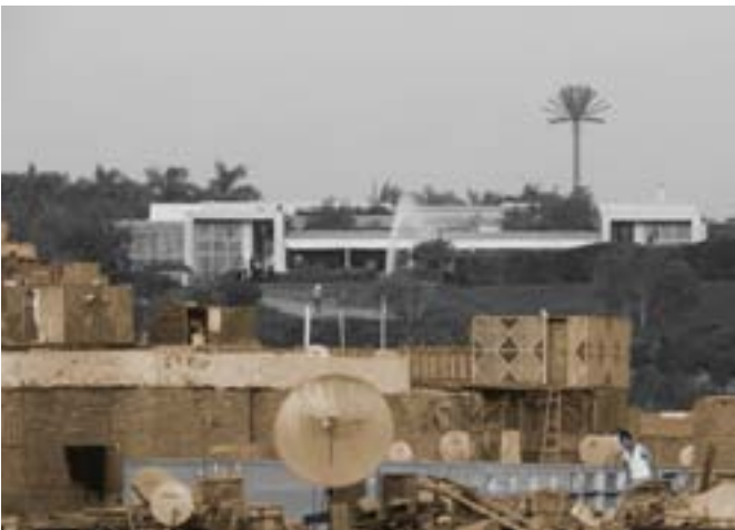
5 Degenerated residential buildings
