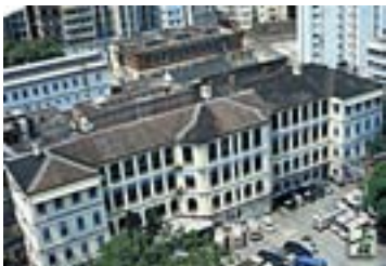
53 Central Police Station Compound deklariert 1995
