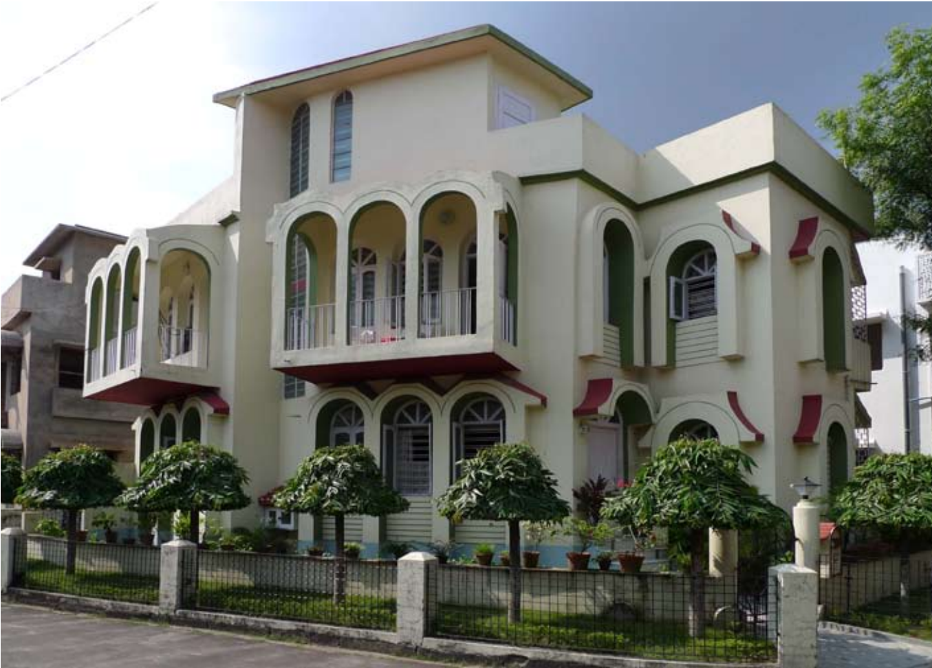
Corner House in AL-Block
