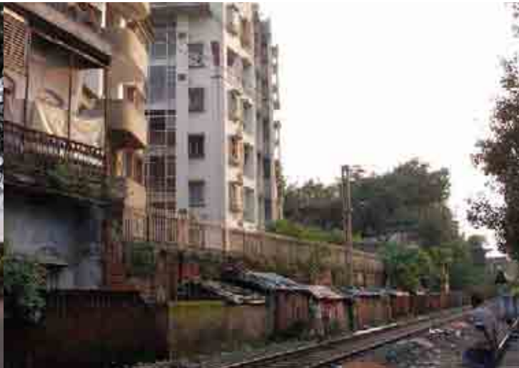
Slum settlement next to the railway
