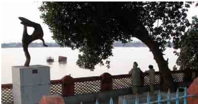
Renovation of the Outram ghat region
