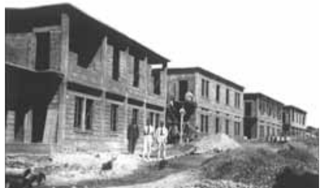
Construction of the "Pavillons blanches"
