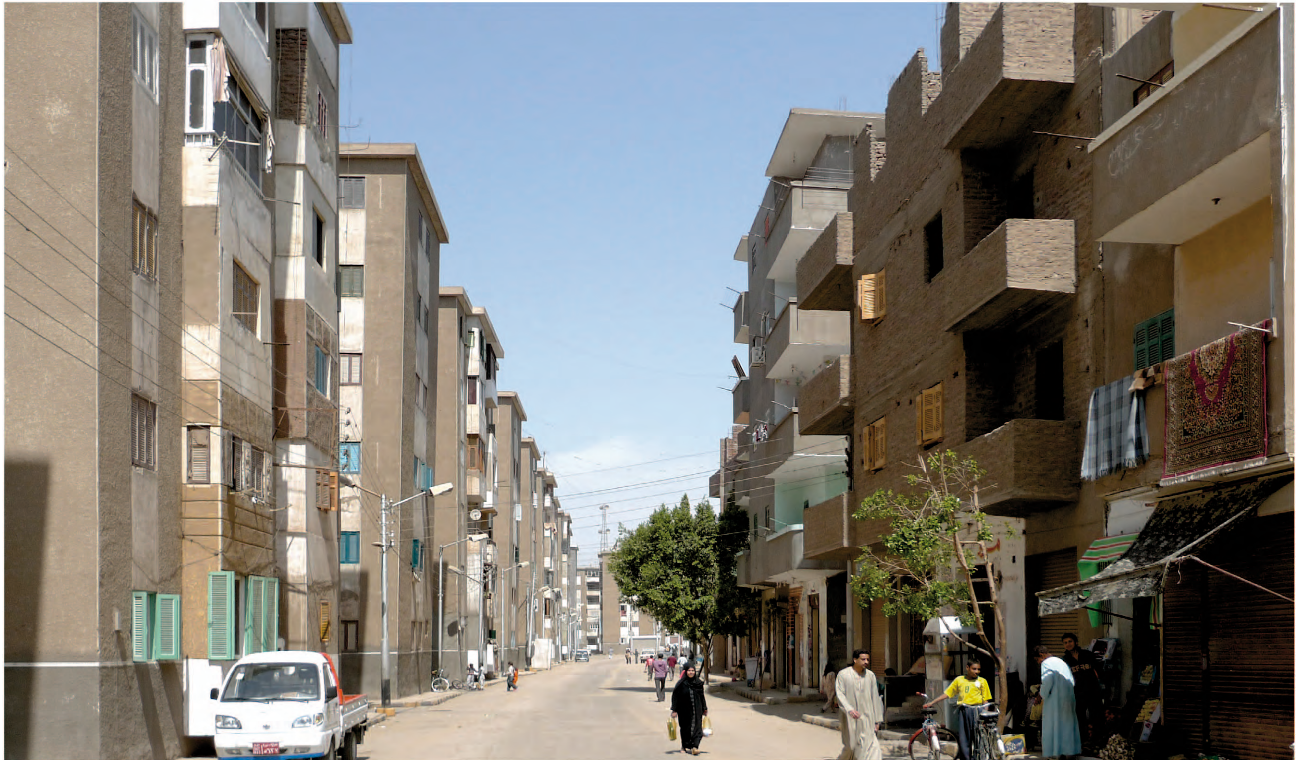
Decaying Public Housing
