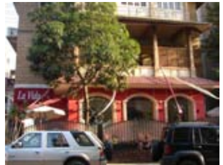
first floor renovation of a restaurant
