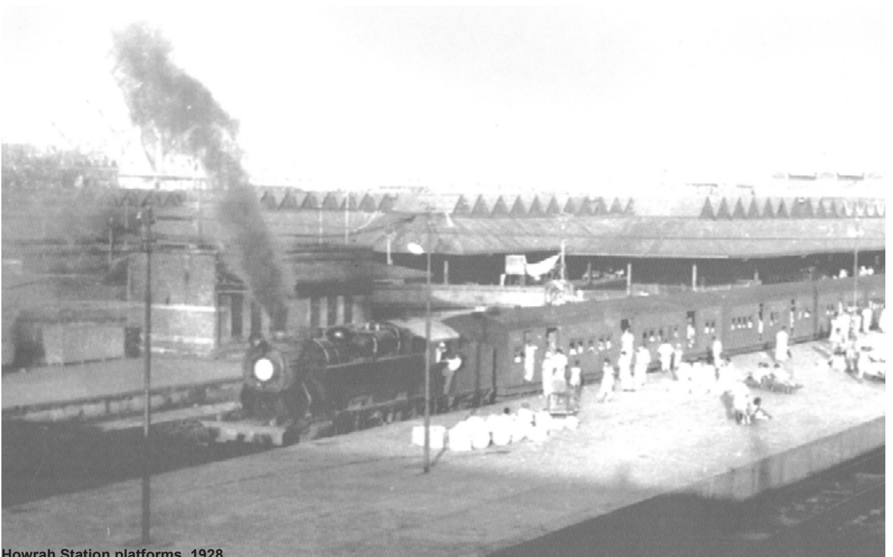
Howrah Station platforms, 1928
