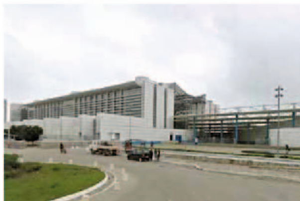
Service (new court house, Pescara)
