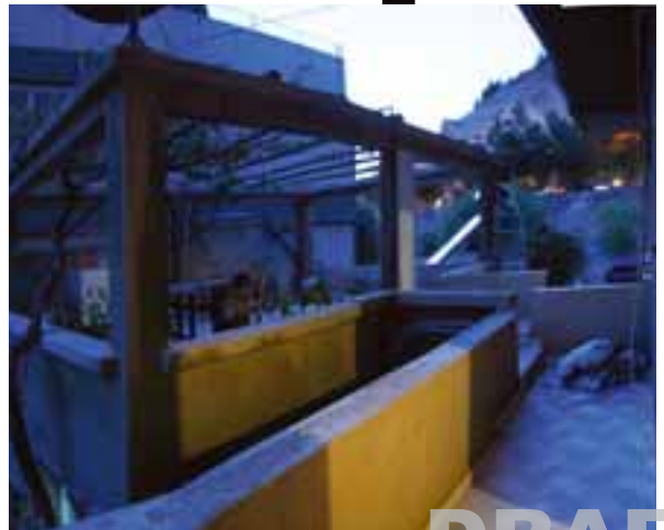
Illegally constructed terrace.
