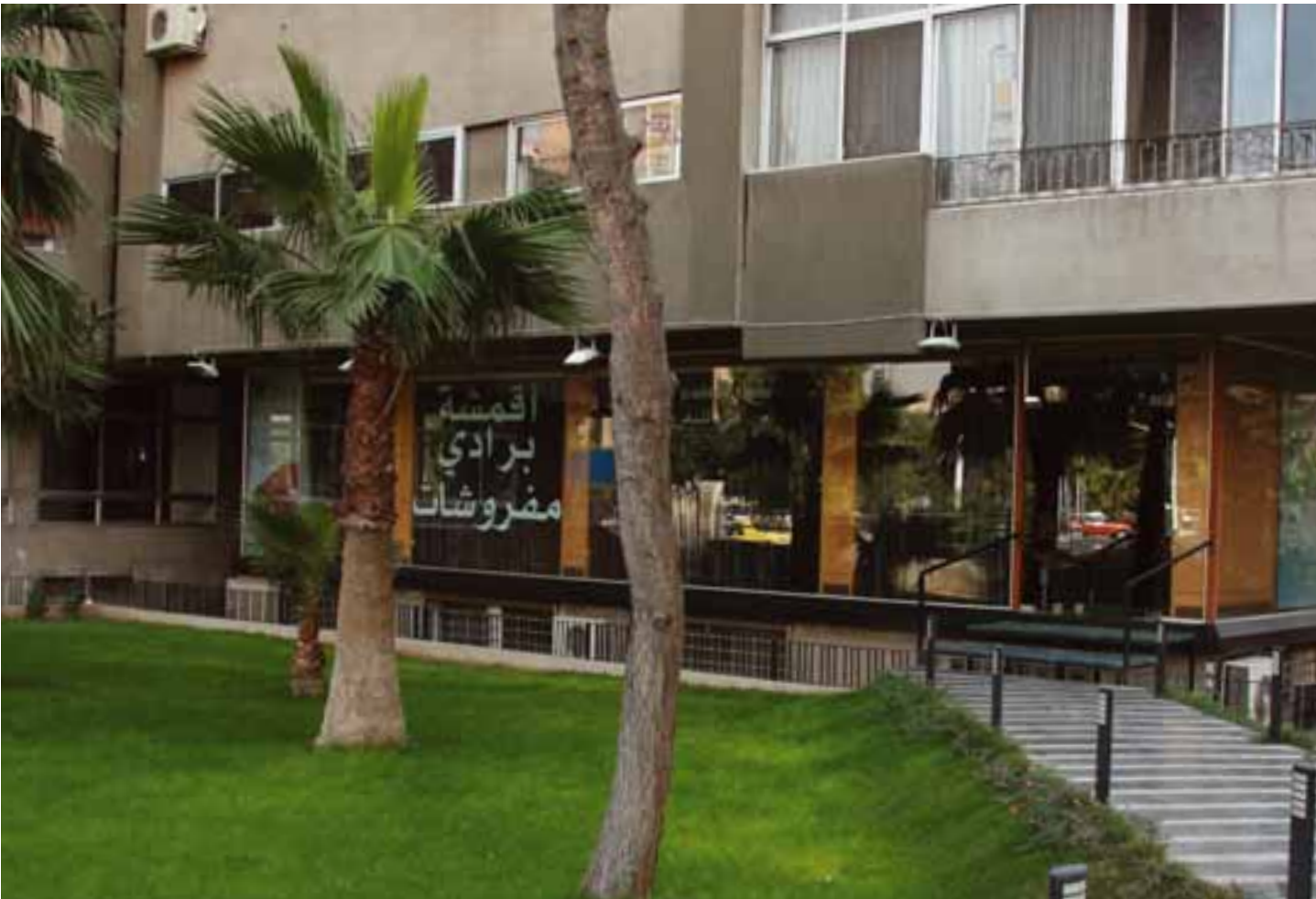
Commercial additions_Rebuilt ground floor
