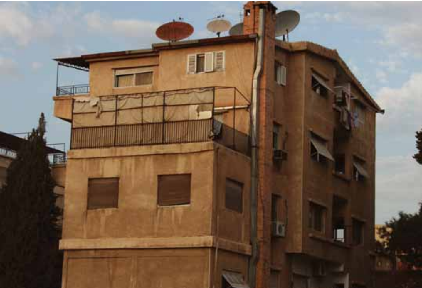
Residential Typologies_Villat_Three illegal additional construction on top of each other
