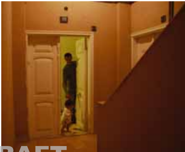
Exterior corridor with 2 entrances for one apartment: one for family, one for guests.
