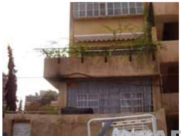
Renovated terrace from the outside.
