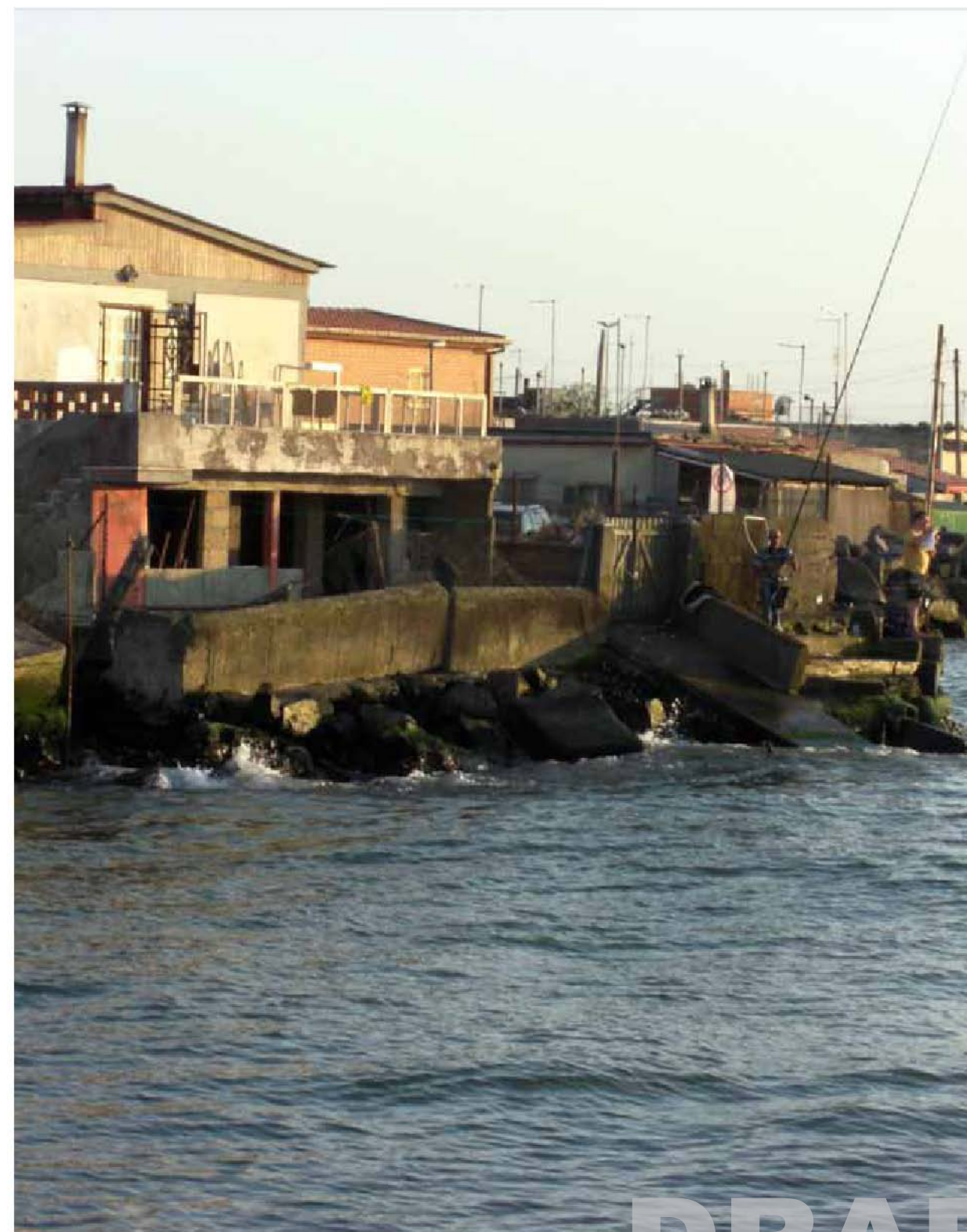
Rock barrier of canal Grande Fiumara
