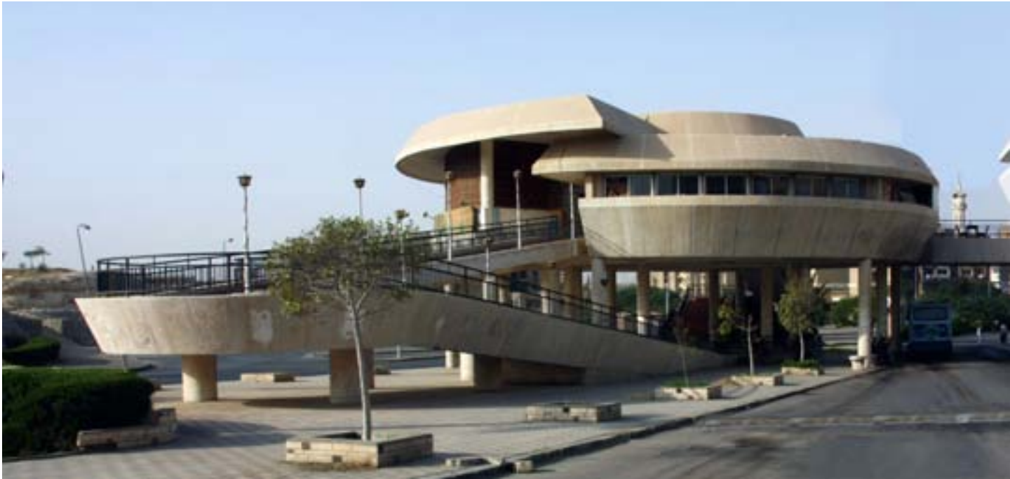
From left to right: Café, Bus station, Parking Garage (not in use) and above the bus station Administration of Statistics of the Helwan Governate
