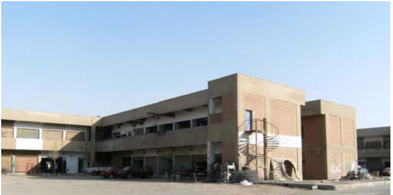
One of the older buildings with garages inside
