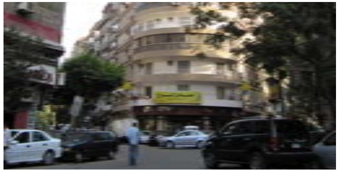
Modern apartments on Zamalek
