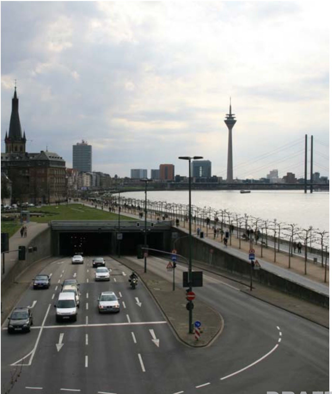
Traffic tunnel to clear the Rhine banks
