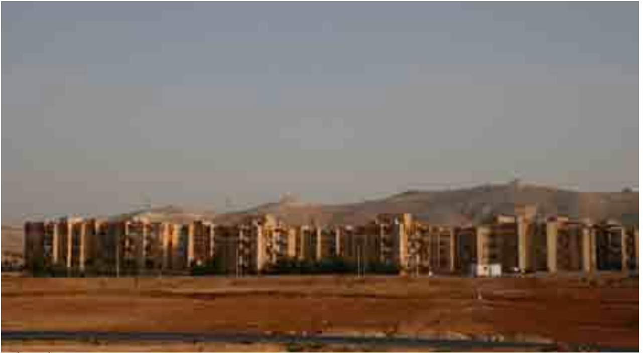
Military housing projects next to site
