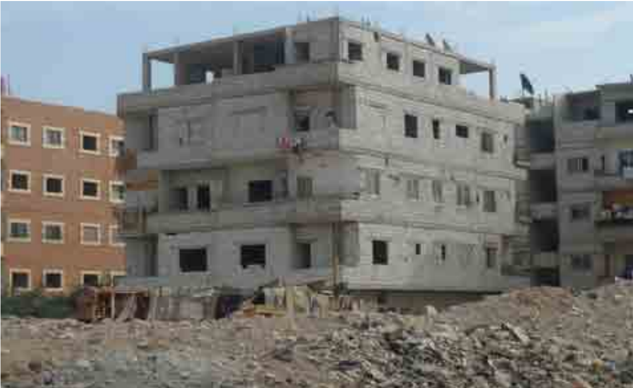
Jaramana housing constructions
