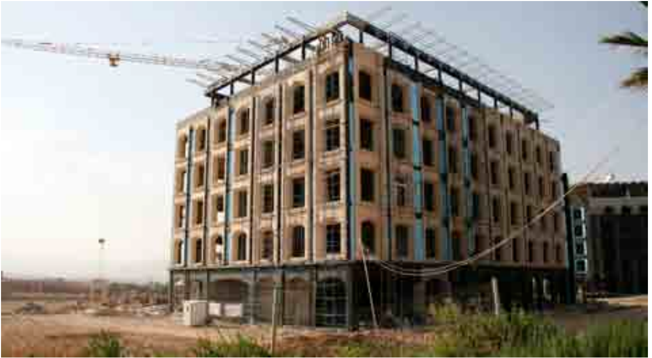
Office building about to be completed
