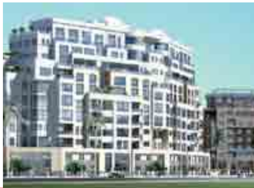
Gated community mixed project in construction
