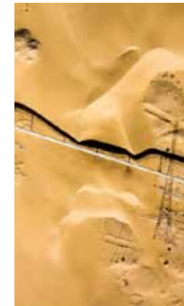
Transportation pipe for phosphate from Bu Craa to the harbour of El Aaiún (100km)
