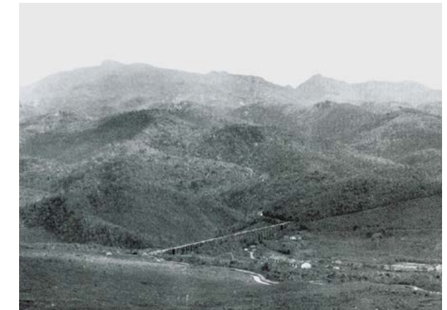
Bicamente aqueduct, water supply for the mine
