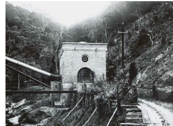
Machina dos Cristais, pump station
