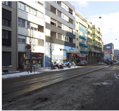
Residential Buildings 1960s-1980s
