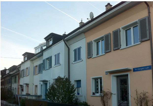
5 Row houses in Im Langen Loh street
