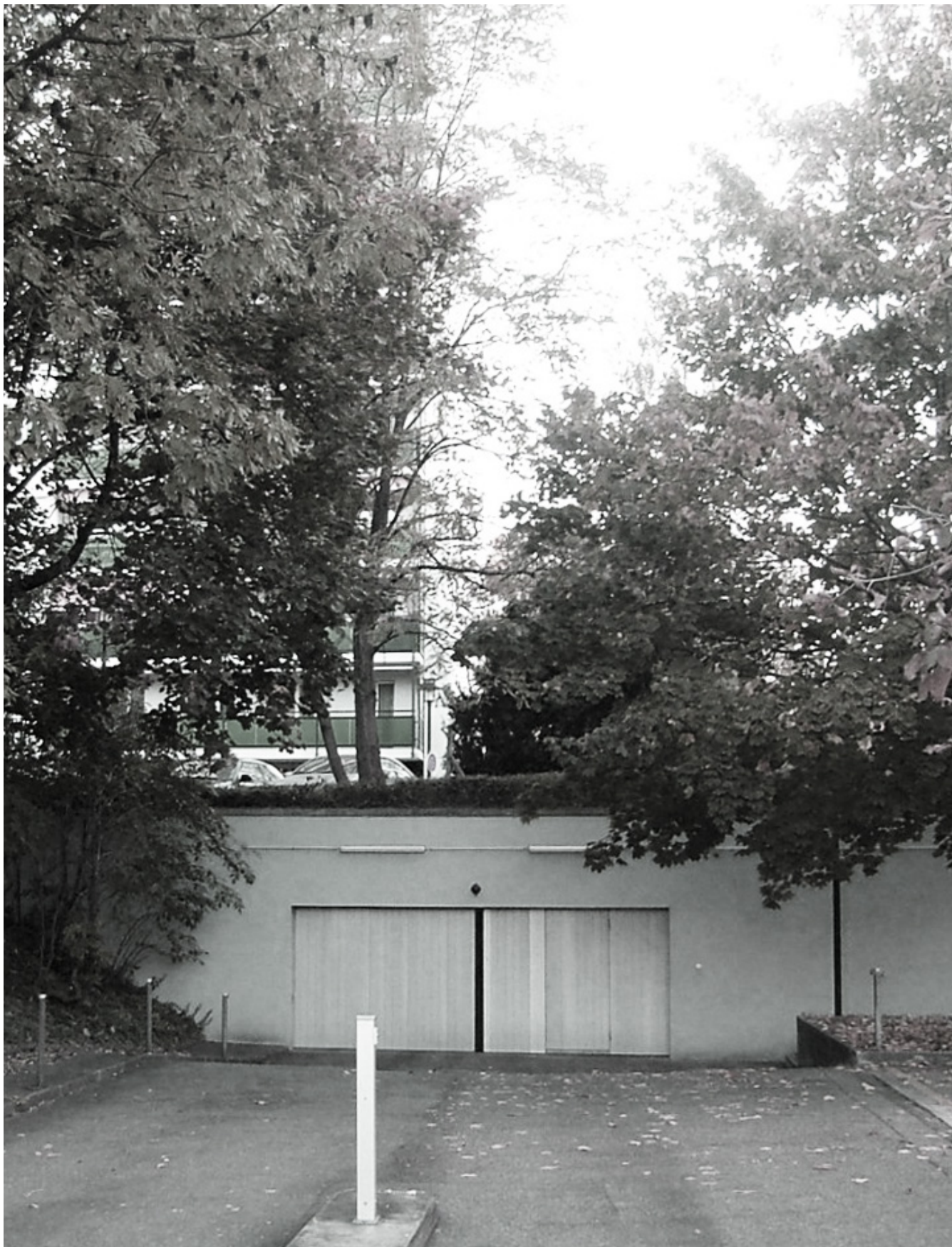
underground garage entrance
