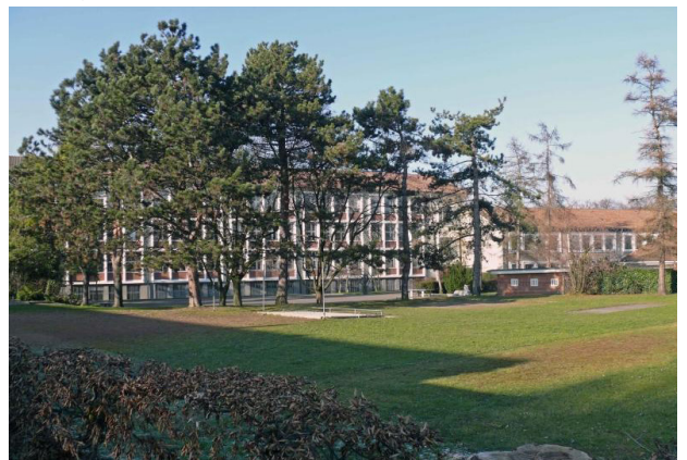
8 Gellertquarter - school building *
