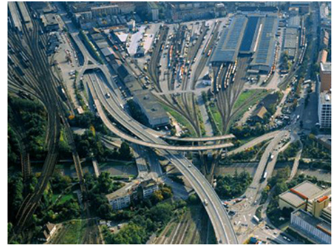
Good Station, North ring road in construction 1995 (www.erlenmatt-ost.ch)
