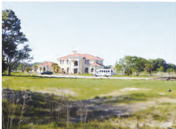
Residential building right beside the preserves boundary
