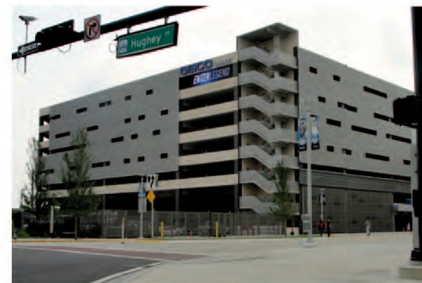
New parking garage
