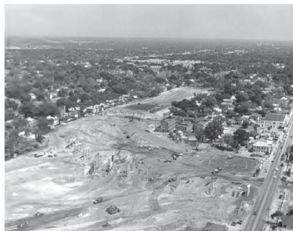
Building I-75 in Tampa, 1963 Construction of an intersection for I-75 near Tampa. With the increased traffic flow, the city needed major connections to highways. Since the residential developments were already built, they were cut by the road.
