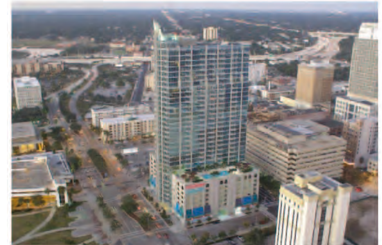
Skypoint Residential Development Courtesy of Metro Jacksonville
