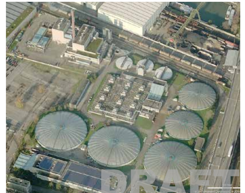
Water Treatment Plant Pro Rheno/Kleinhüningen BS (Aerial Photo/Bing Maps)
