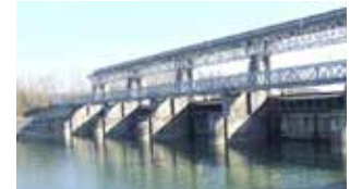
Dam at the Kembs Powerplant, Canal d'Alsace, France
