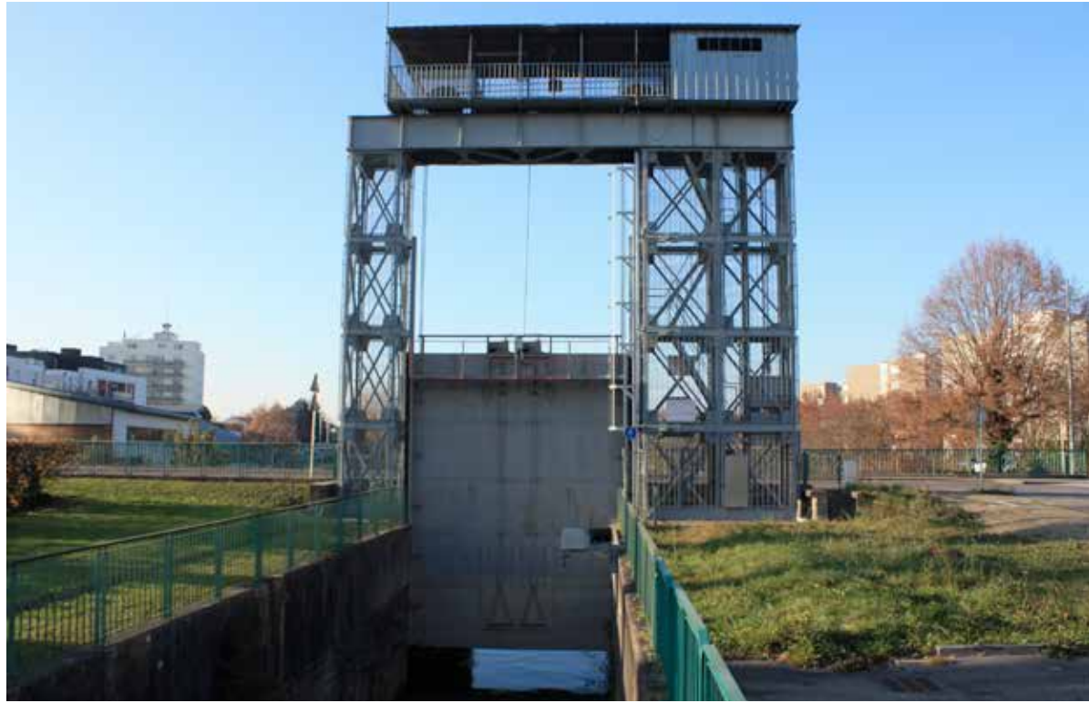
The locks at Canal de'Huningue/F are no longer operational
