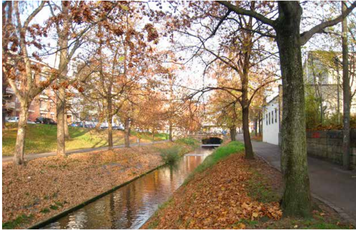
Transition from open river to and underground canal, the River Birsig in Basel City
