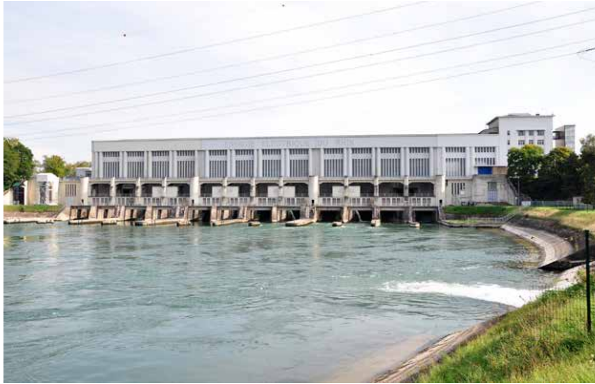
Power Plant Kembs, France ( http://www.panoramio.com/photo/41190246 )
