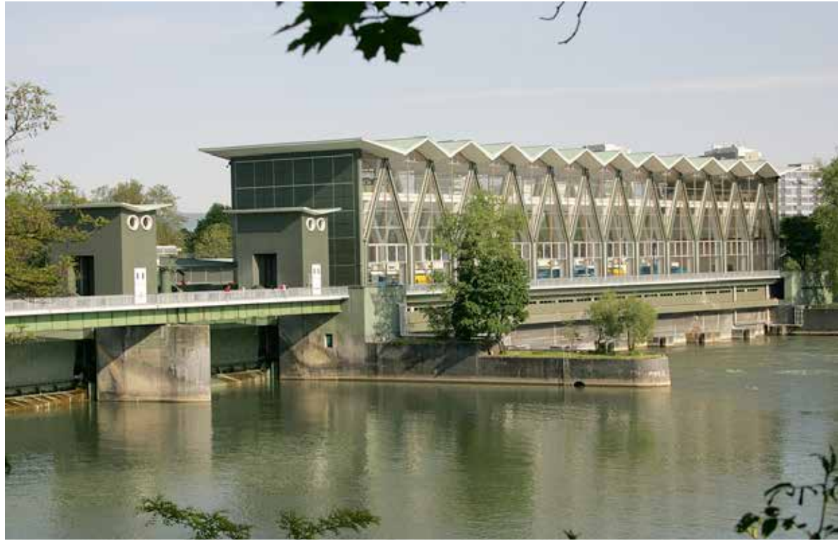
Hydroelectricity Plant Birsfelden/BL
