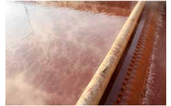
ARA Pro Rheno Basel/5. Sludge Basin
