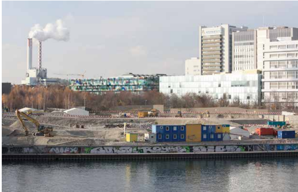
The Novartis Campus from Dreilaenderbrücke
