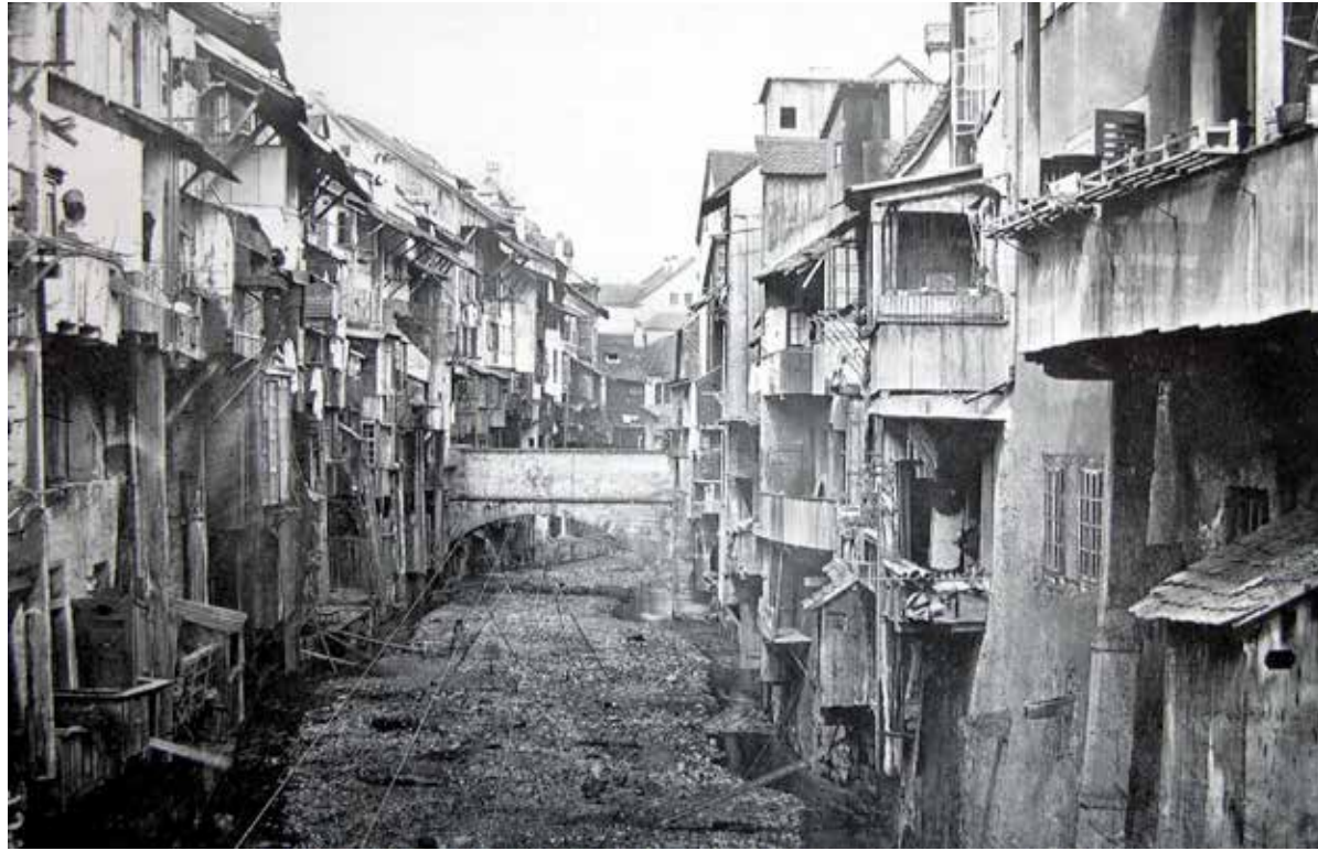
Historical photo of the river Birsig before rehabilitation
