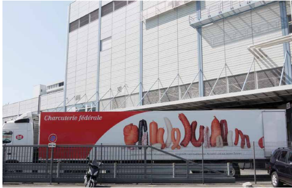
Bell Group processing plant in Basel.
