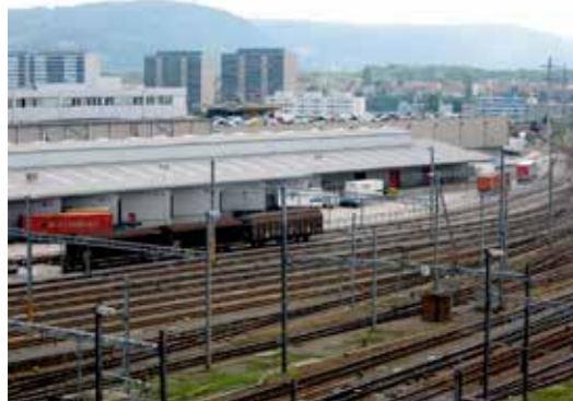
Freight handling station Wolf, UAG ( http://www.homegate.ch )
