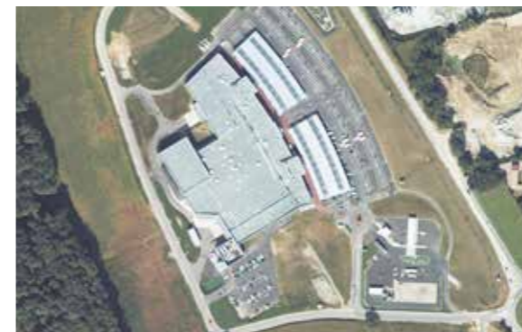
Partially roofed parking and entrance
