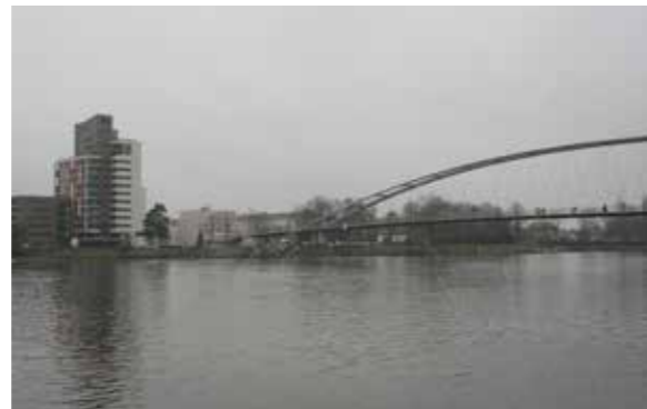
Pedestrian bridge connecting Huningue and the Rhein Centre
