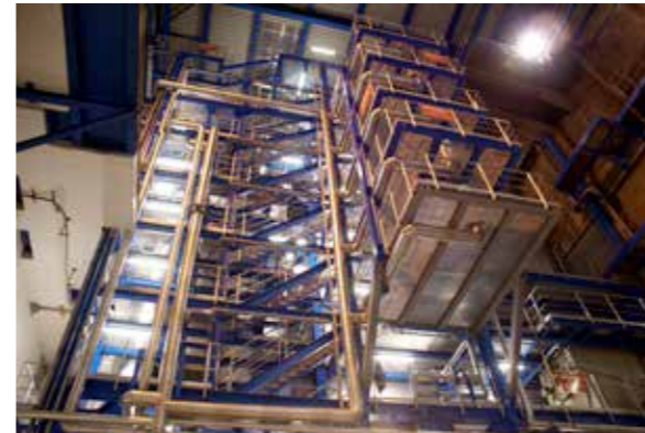
(13) electrostatic precipitator (filter)
