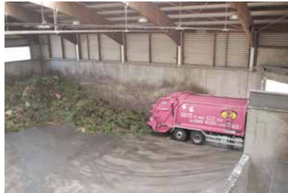
(3) Large reception hall for waste
