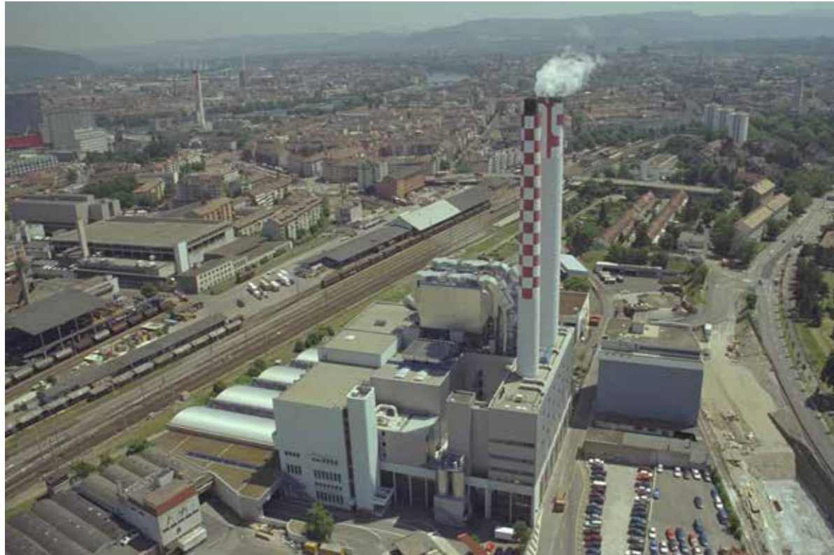
KVA Basel source: IWB
