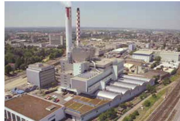
(15) chimney / standby chimney
