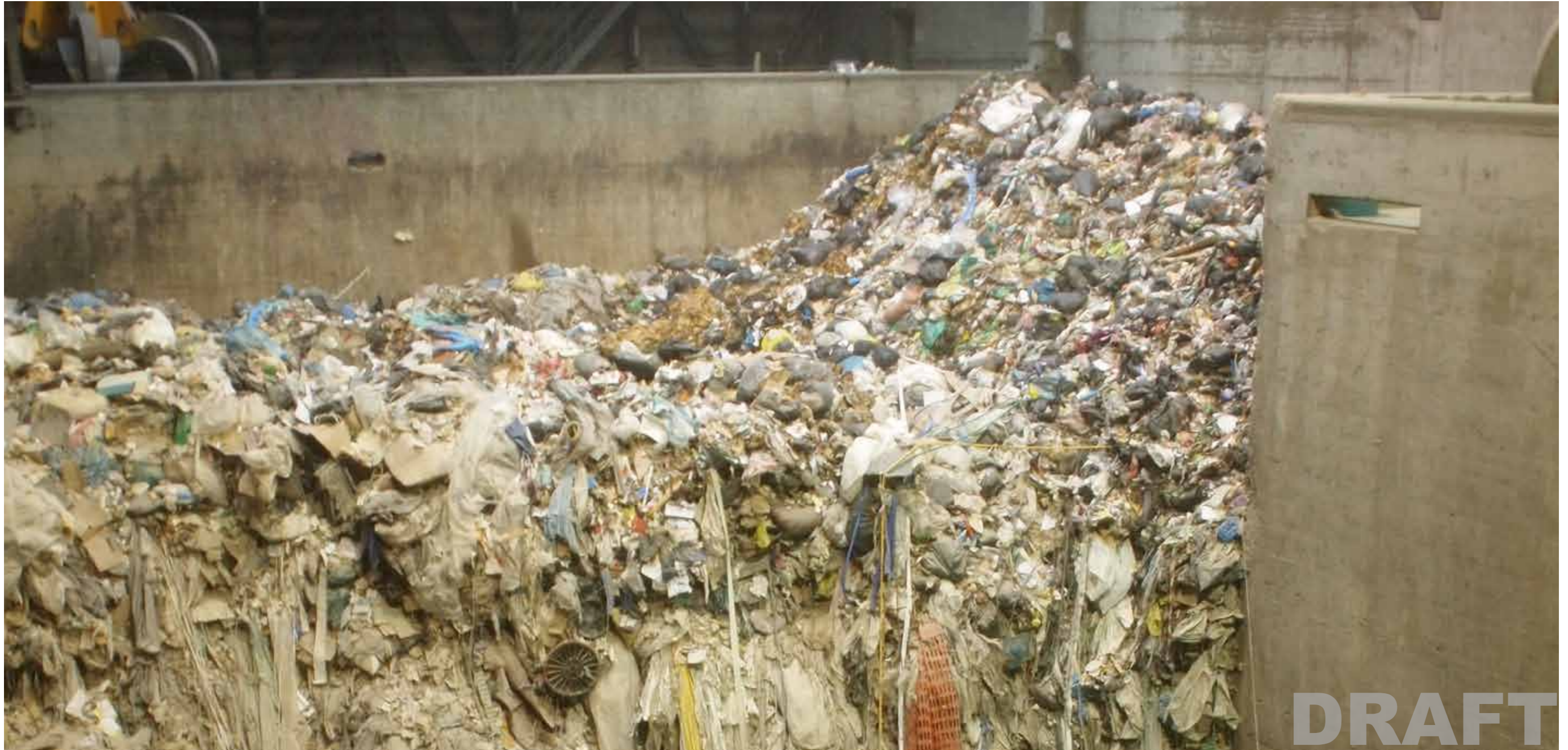
Waste bunker at the incineration plant, Basel
