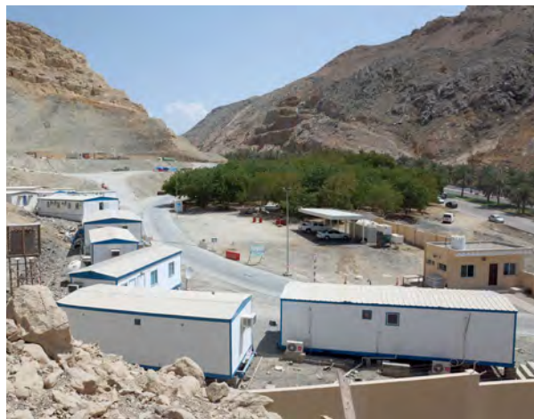
Construction site of the mudflowdam
